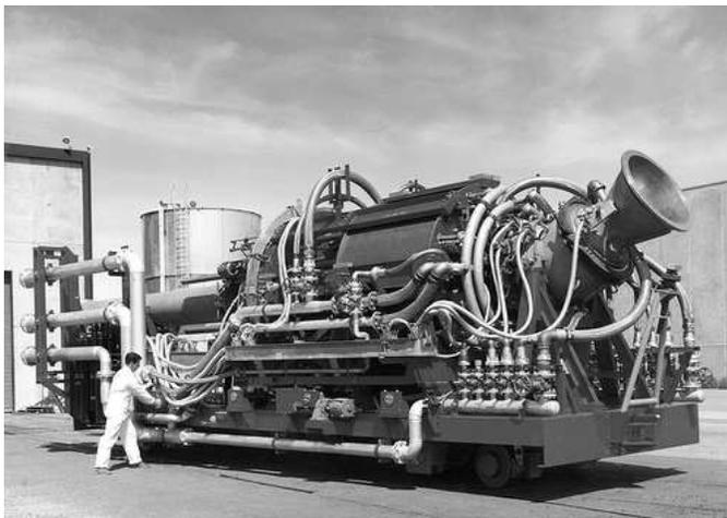
Their purpose was solely to demonstrate feasibility of design. Weighing over a hundred thousand pounds, each, they were built on railcars to facilitate movement to remote test locations. After each test, the reactor's railcar would be returned to a heavily shielded maintenance bay for disassembly & analysis. Their size can best be appreciated when viewing this photo.
