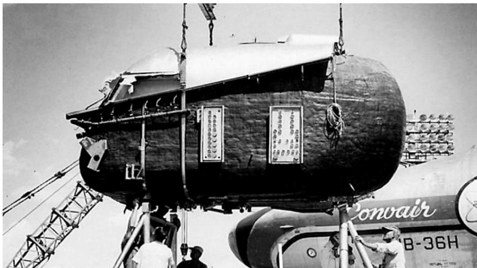
Between July 1955 and March 1957, the NB-36H flew forty-seven flights. On several of these flights, the reactor was operated up to a power level of three megawatts. Despite persistent rumors to the contrary, the test aircraft was not powered by the reactor it carried. The sole purpose of those flights was to gather data useful for future shielding design of an actual nuclear-powered aircraft.
