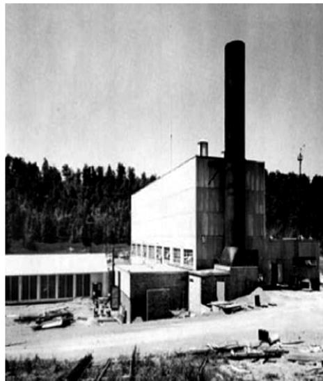
The first test run of the Aircraft Reactor Experiment took place in October 1954. The reactor ran at a power level of one mega-watt for 100 hours. The design and construction of such an exotic device in less than five years was considered a noteworthy achievement.
