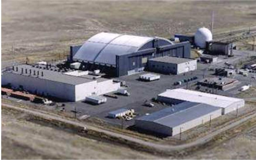
This hangar was equipped with thick walls for shielding and plans were made to enable extraction of an aircraft's reactor and place it in a shielded storage bay using remote control methodology. Included in these never-realized plans, were closed-circuit television systems and remote manipulator arms to allow technicians to work on the aircraft & its power plant without direct exposure to the intense radiation fields that would exist even shortly after reactor shut down.
