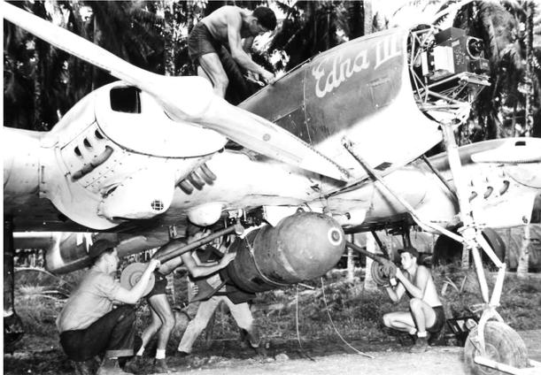
The photo on the left, probably posed, shows ground crews preparing a TDR-1 for action. Their scant attire indicates the high heat and humidity conditions which they faced. Clearly visible is the aircraft's single bomb load. The drone's nose cone, not yet attached, allows for an excellent view of the Block-1 TV system.
